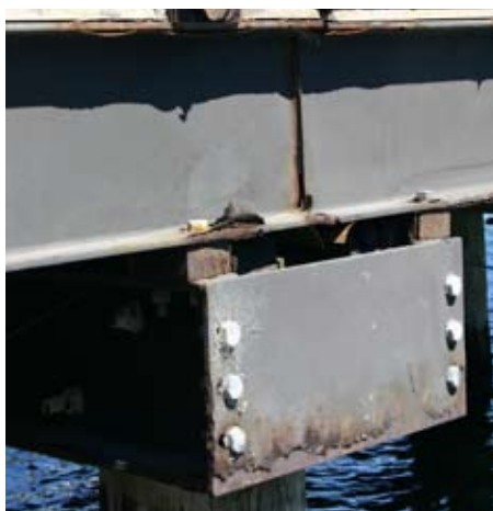
Failing paint coating
